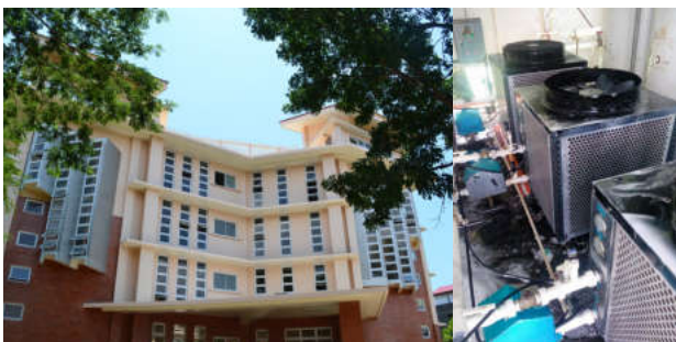
LYCEUM OF THE PHILIPPINES UNIVERSITY (LPU) P. Herrera cor. Dona Aurelia St., Kumintang Ibaba, Batangas City
